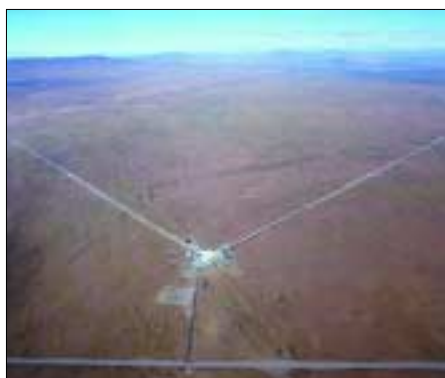
Reaching out – the LIGO facility in the US consists of a pair of laser interferometers that search for tiny changes in the separations of test masses caused by the passage of gravitational waves. Each interferometer – one at Hanford in Washington state (above), the other near Livingston in Louisiana – has arms that are 4 km long.
